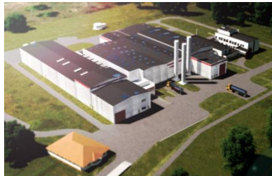
Expansion of Chocolate plant in Lodz Poland
